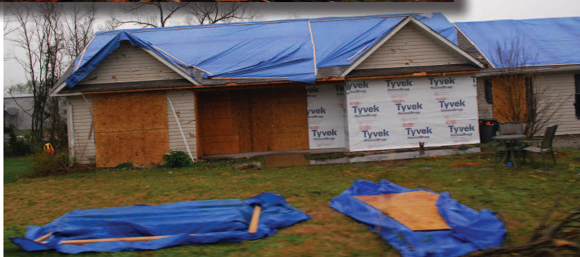
The photos above depict the damage done by a Tornado that ripped through the community of Greenback on March 23rd of this year. The National Weather Service determined that the tornado was an EF 3. The storms that plowed through Blount County on April 27th produced several tornadoes, one of which was declared an EF 4 with wind speeds of over 170 mph. (Photos by Tech. Sgt. Kendra M. Owenby, 134 ARW Public Affairs)
