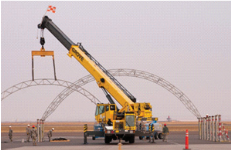
Members of the 134th Civil Engineering Squadron from McGhee Tyson Air National Guard Base, Tenn. and members of the 819th RED HORSE Squadron from Malmstrom Air Force Base use a hydraulic crane to dismantle an aircraft inclement weather shelter at the 120th Fighter Wing on Sept. 14, 2012. The Tennessee Air National Guard Airmen deployed to Montana to conduct their deployed field training. (National Guard Photo by Staff Sgt. Scott Hollis)
