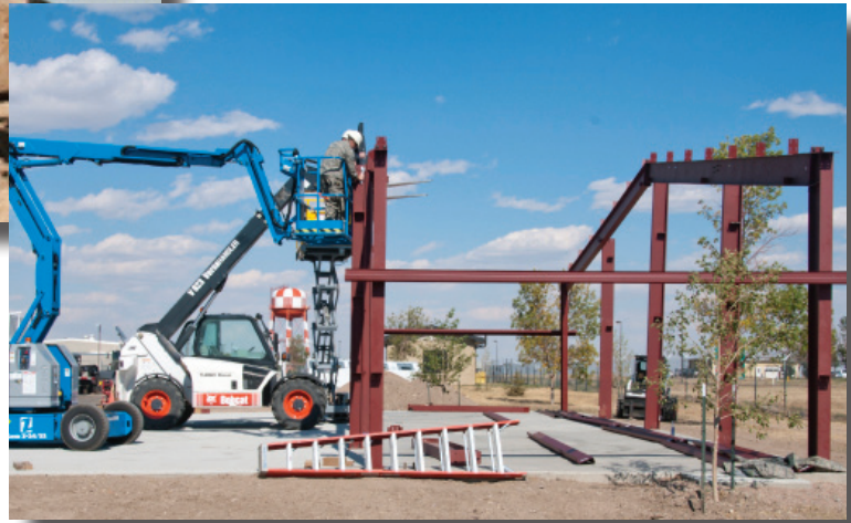
Senior Airman Kyle J. Paridee (above) of the 134th Civil Engineering Squadron uses a front-end loader to remove a concrete pillar that had held a former static display at the 120th Fighter Wing, Great Falls ANG Base, Montana. Members use a lift (right) to assist them in constructing a pre-fabricated metal building to be used as a recycling center for the 120th FW. The building was constructed on a pre-existing concrete foundation. (National Guard Photo by Staff Sgt. Scott Hollis)
