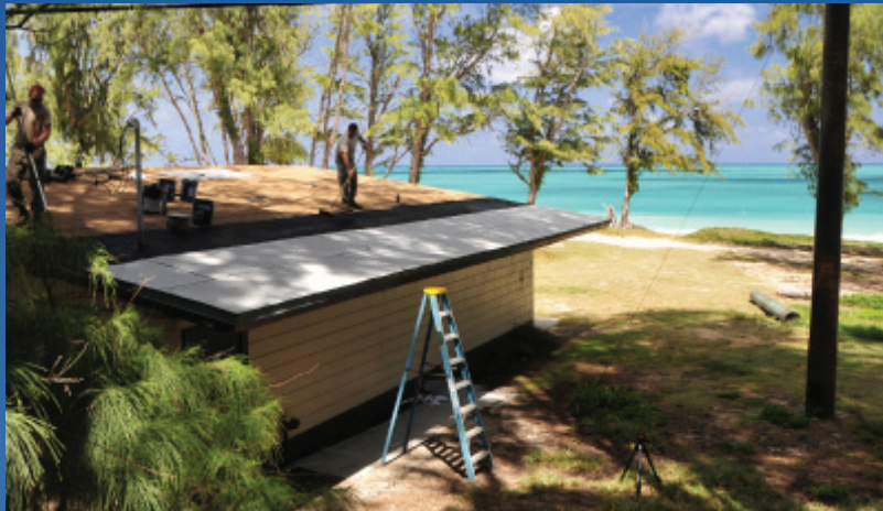
Airmen First Class William Frosell and John Mason, (above), apply tar to the roof of a building. Senior Airman Henry Queen, drills holes for copper piping to be installed. The 134 ARW Civil Engineer Squadron members completed several projects during their Deployed Field Training to Bellows Air Force Station Aug 3-18. (U.S. Air National Guard photo by Master Sgt. Kendra M. Owenby, 134 ARW Public Affairs)
