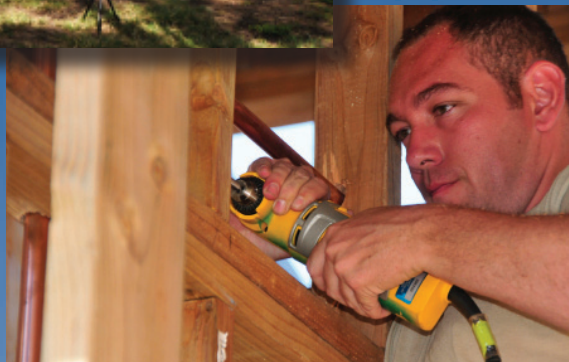
Airmen First Class William Frosell and John Mason, (above), apply tar to the roof of a building. Senior Airman Henry Queen, drills holes for copper piping to be installed. The 134 ARW Civil Engineer Squadron members completed several projects during their Deployed Field Training to Bellows Air Force Station Aug 3-18. (U.S. Air National Guard photo by Master Sgt. Kendra M. Owenby, 134 ARW Public Affairs)
