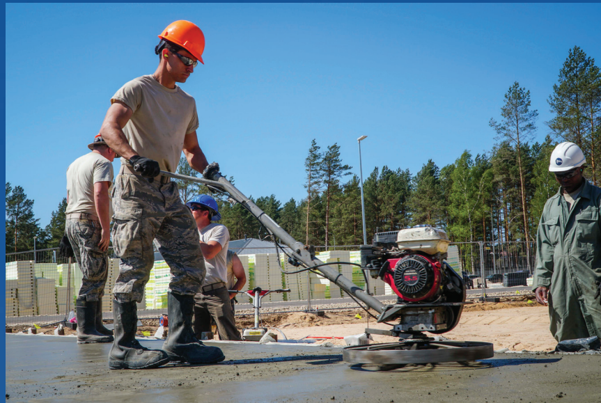
Airmen from the 134th Civil Engineer Squadron construct concrete pads during their annual deployment for training May 4-19 at Camp Adazi, Latvia. (U.S. Air National Guard photo by Staff Sgt. Ben Mellon)
